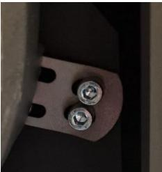
5. Remove the smoke exhaust fan by first cutting the silicone around the pipe, then pull the smoke exhaust fan down and pull it outwards:
