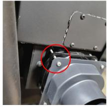
5. Connect the Air Booster to the two free slots in the white electric socket for the fans, one in each slot marked N and L:
