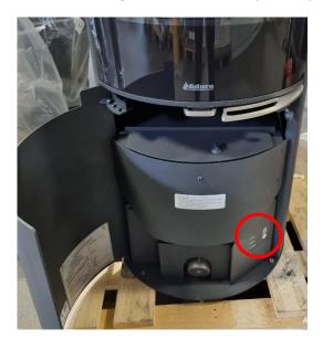
2. The control panel is glued onto the surface of a cover plate (on some newer models the control panel is placed in a recess in the plate). Take note of the orientation of the cable connected to the control panel. To remove the control panel, use a small flathead screwdriver/a Stanley knife to lift the control panel off the surface. Be careful! This might break the control panel.
