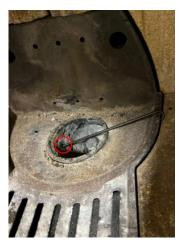
When the ceramic ignitor has been placed properly, connect the cables to the socket (the blue cable in one of the "N" holes and the red/brown cable in one of the "L" holes):
